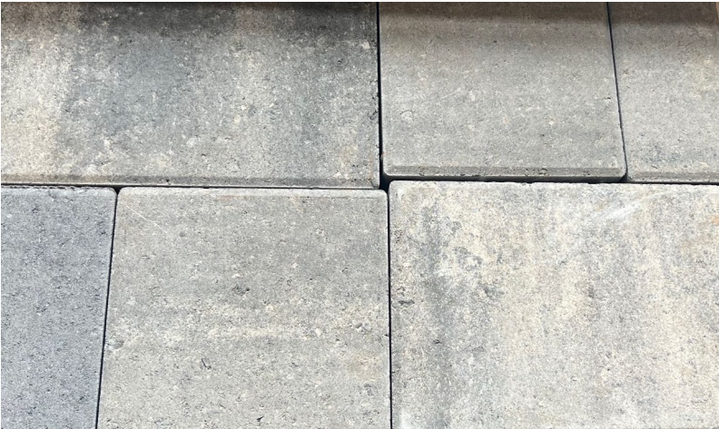
Basement Patio Paver
