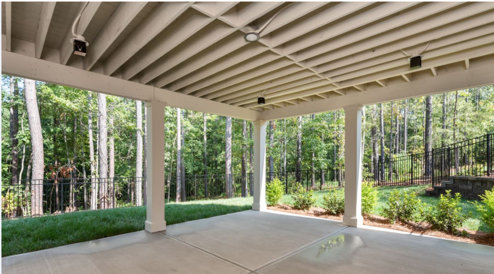
Ceiling Fan Pre-Wire Under Deck With Additional Lighting
